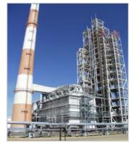
Catalytic reformer with continuous catalyst regeneration — 1 mln tons per year
