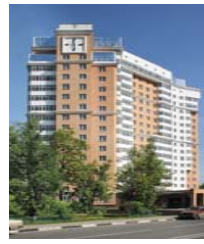
Presnya House, Moscow, 16k m 2 , 2007
